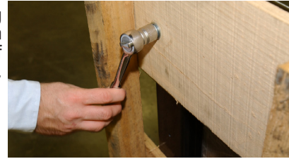
Removing skid from bottom of cabinet.
