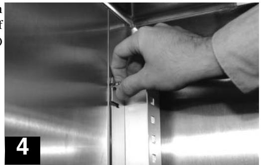
Pilaster Installation (Side Wall of Cabinet)
