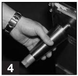
Thread leg into cabinet bottom frame rail.
